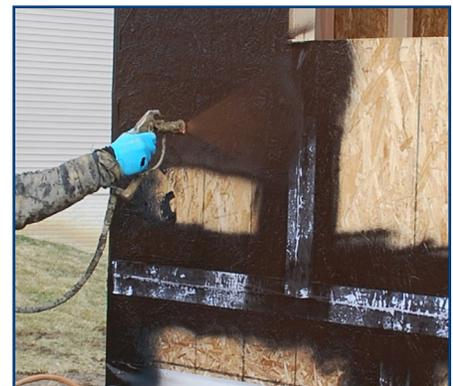
Seals sheathing joints, preventing air and water infiltration & damage.
