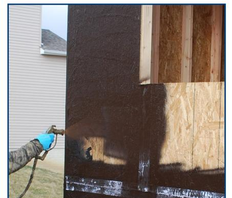
Uniformly coats and protects sheathing from liquid moisture penetration, but allows vapor to escape.
